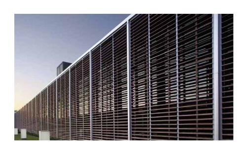
Due to the southern position of the facade of the commercial establishment is intended to protect through louvers, these louvers will be an integral part of the composition of the same. In addition to protecting, the parasole will be able to sift the internal light during the night.
